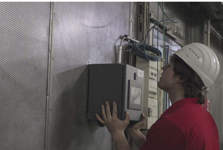
Using a separately installed server, the data are transmitted directly from the sensor without connecting to the company network
